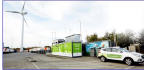
COLRUYT GROUP Water electrolysis | Belgium The pilot of the retailer Colruyt Group produces Green Hydrogen with electrolysis for their forklifts, heavy duty vehicles and passenger cars.
