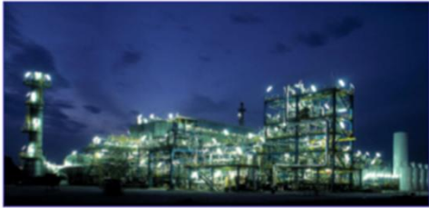
SMR Port Jerome | France The pilot plant by Air Liquide produces Low Carbon hydrogen using steam methane reforming with a Carbon Capture unit or Green Hydrogen using BioMethane as feed gas.
