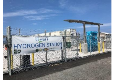
Hydrogen station at NELHA
