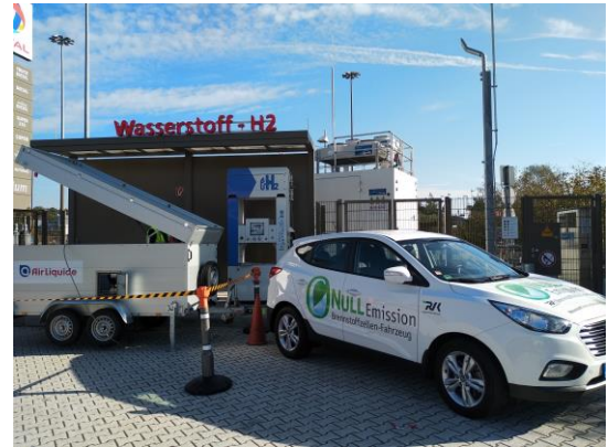
Figure 4: Installation at Cologne HRS
