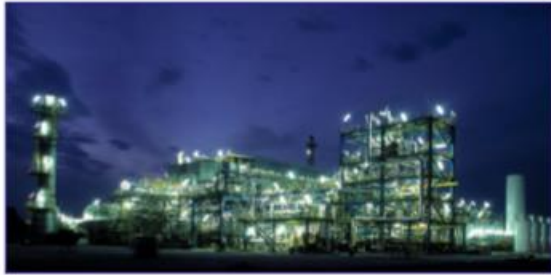
SMR Port Jerome | France The pilot plant by Air Liquide produces Low Carbon hydrogen using steam methane reforming with a Carbon Capture unit or Green Hydrogen using BioMethane as feed gas.
