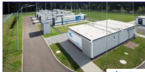
Windgas Falkenhagen | Germany The pilot by Uniper produces Green Hydrogen from wind energy via water electrolysis, that can be fed into the natural gas grid or used as input for methanation.
