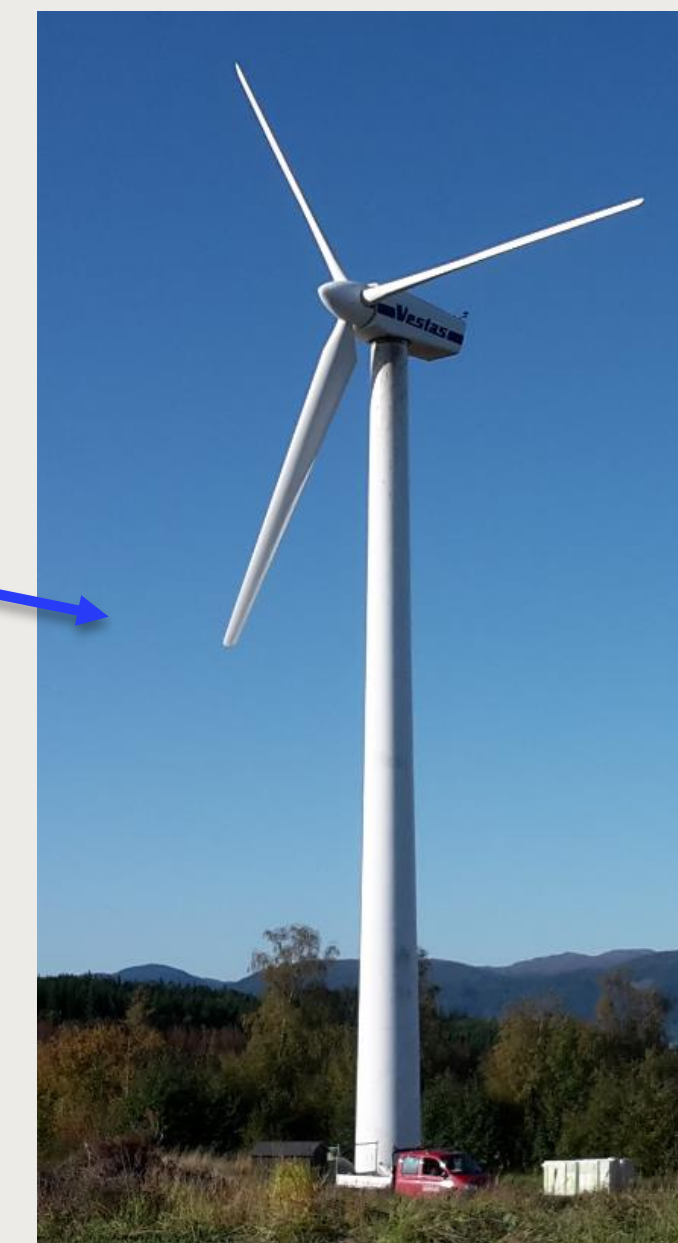
225kW Wind turbine
