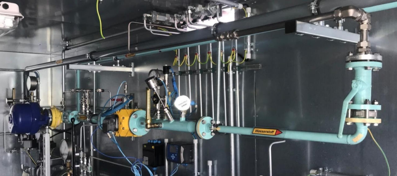
The pressure is reduced to 10 bar at the electrolysis system before the outlet
