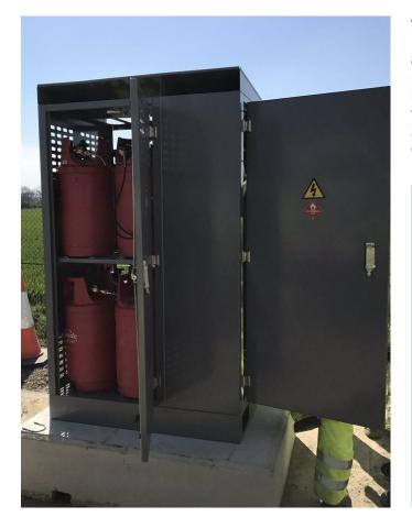
**Brief description:** stationary fuel cells for off-grid or isolated microgrids provide base-load (or backup) electricity from hydrogen (or hydrocarbons) via a fuel cel); fuel cells are frequently combined with electrolyzers for power-2-hydrogen from renewables – as integrated end-to-end off-grid solutions
