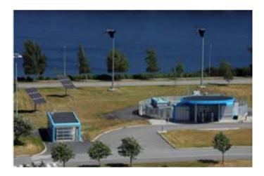
Figure 1: Statoils Energy Park at Herøya, Porsgrunn, Norway. The energy park consists of two 6 kW wind turbines and two 2.1kW solar panels and is equipped with a 70 kWh lead acid battery storage system, and water electrolysers from NEL Hydrogen (Earlier Hydrogen Technologies).
