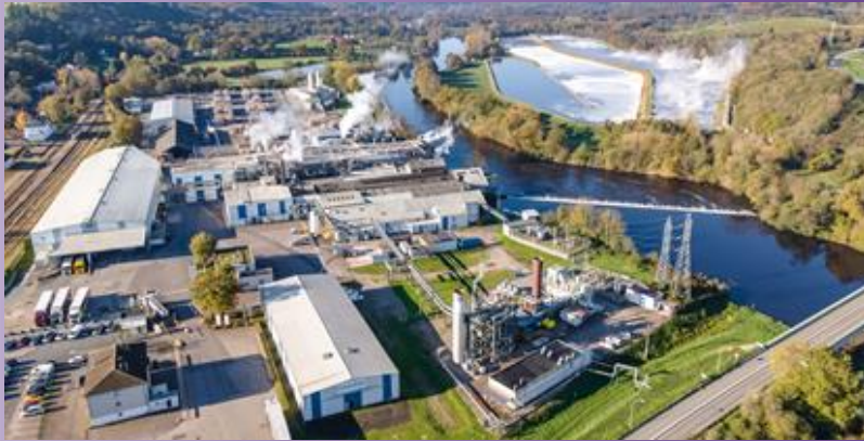
Smurfit Westrock SGT-400 Cogeneration Plant Saillat-sur-Vienne, France
