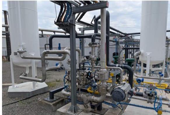
Mixing station with improvements
