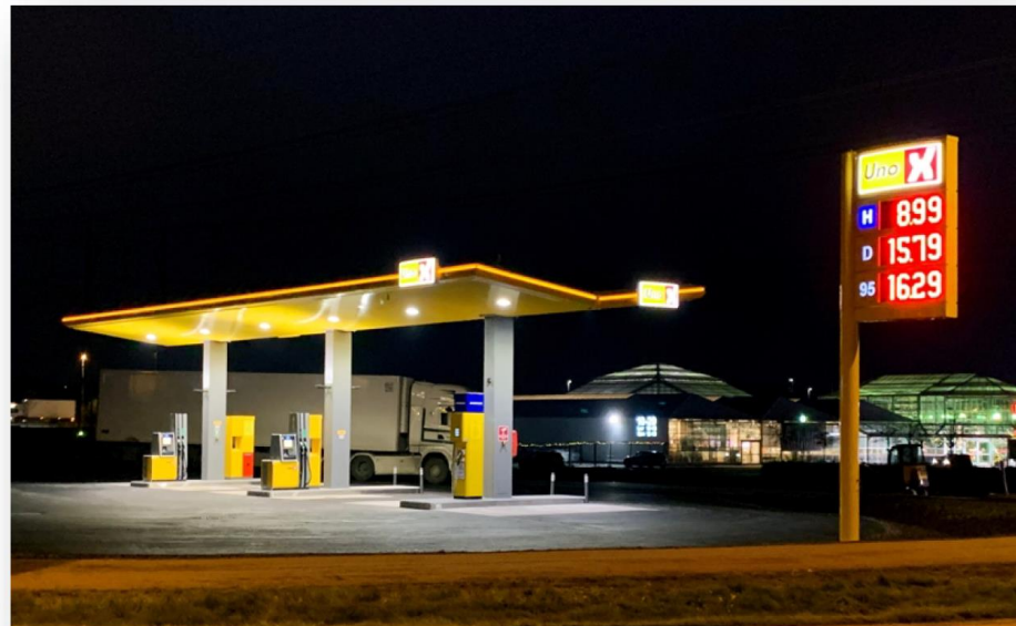
Newly opened energy station at Hvam, Norway (Photo: Uno-X)
