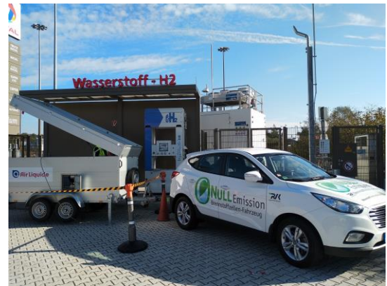
Figure 4: Installation at Cologne HRS
