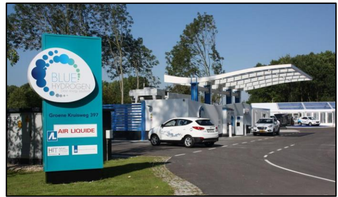
AL station - Rotterdam (Rhoon)
