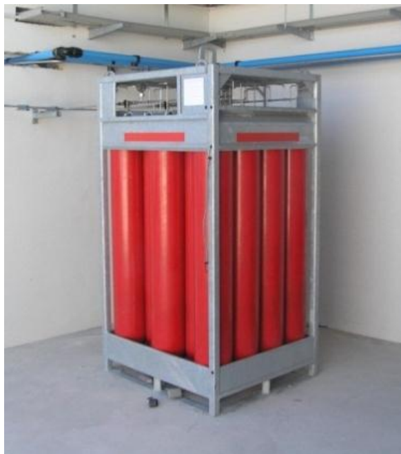
Figure 2.11. High pressure hydrogen storage at 350 bar.
