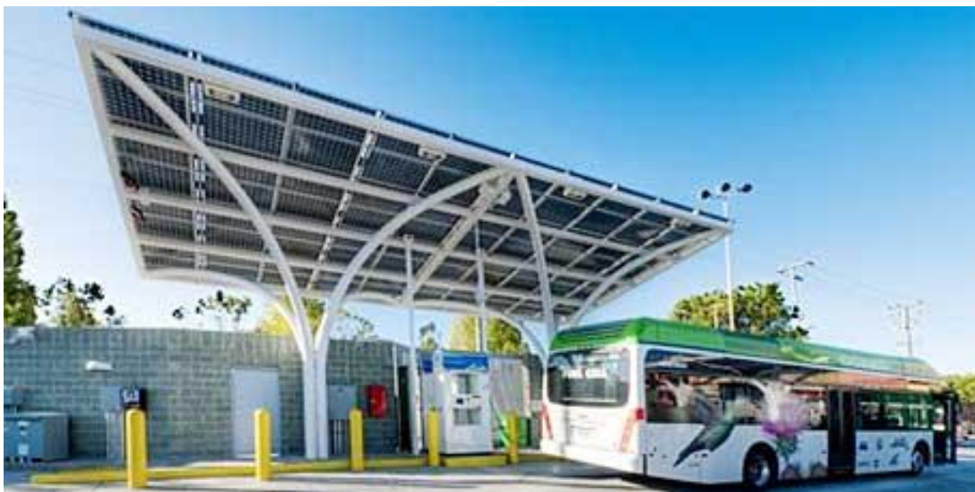
Figure 2.15. Hydrogen filling station of Emeryville (California, USA).
