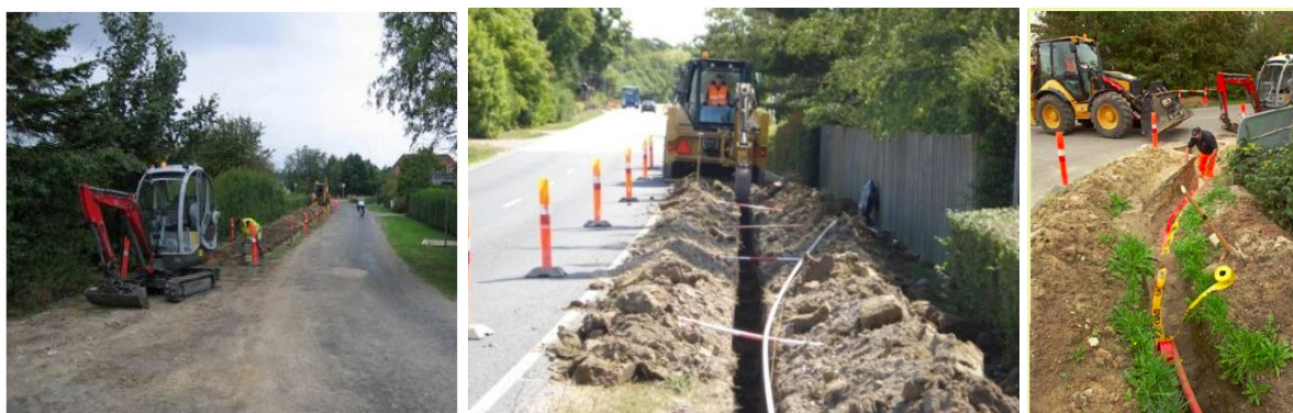
Figure 4.5. Building of the hydrogen grid infrastructure.
