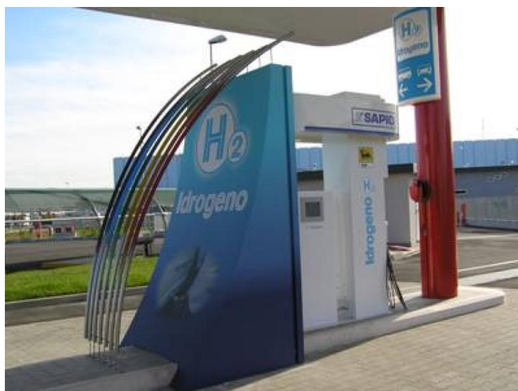
Figure 2.25. 350 bar dispenser in Mantova and concrete wall protection.
