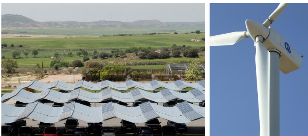
Figure 2.7. The power for hydrogen production comes from solar panels and wind turbine.
