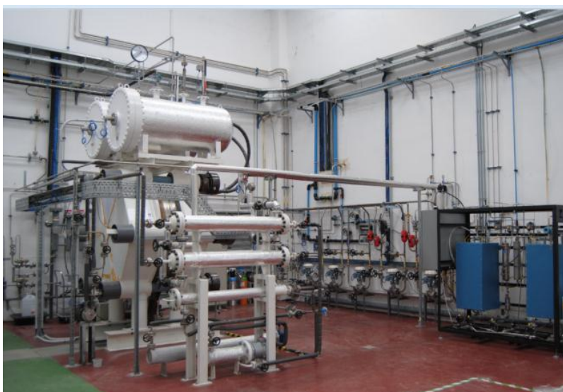
Figure 2.8. Alkaline electrolyzer for hydrogen production.
