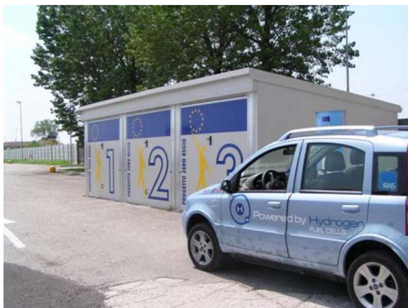
Figure 2.27. Garage for hydrogen vehicles into offices of SAPIO plant.
