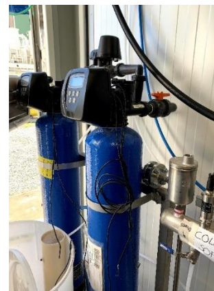
Water Softening System
