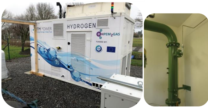
180kW PEM electrolyser and hydrogen injected into the natural gas grid
