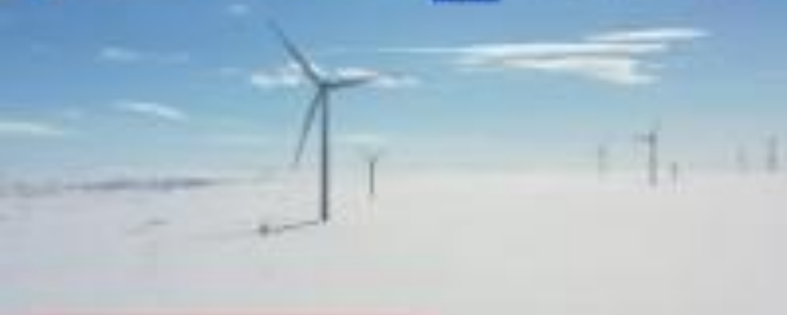
Raggersvolden Wind Farm
