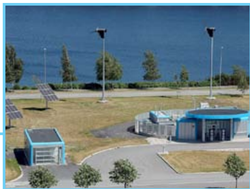
Statoils Energy Park at Herøya, Porsgrunn, Norway. The energy park consists of two 6 kW wind turbines and two 2.1kW solar panels and is equipped with a 70 kWh lead acid battery storage system, and water electrolysers from NEL Hydrogen (Earlier Hydrogen Technologies).
